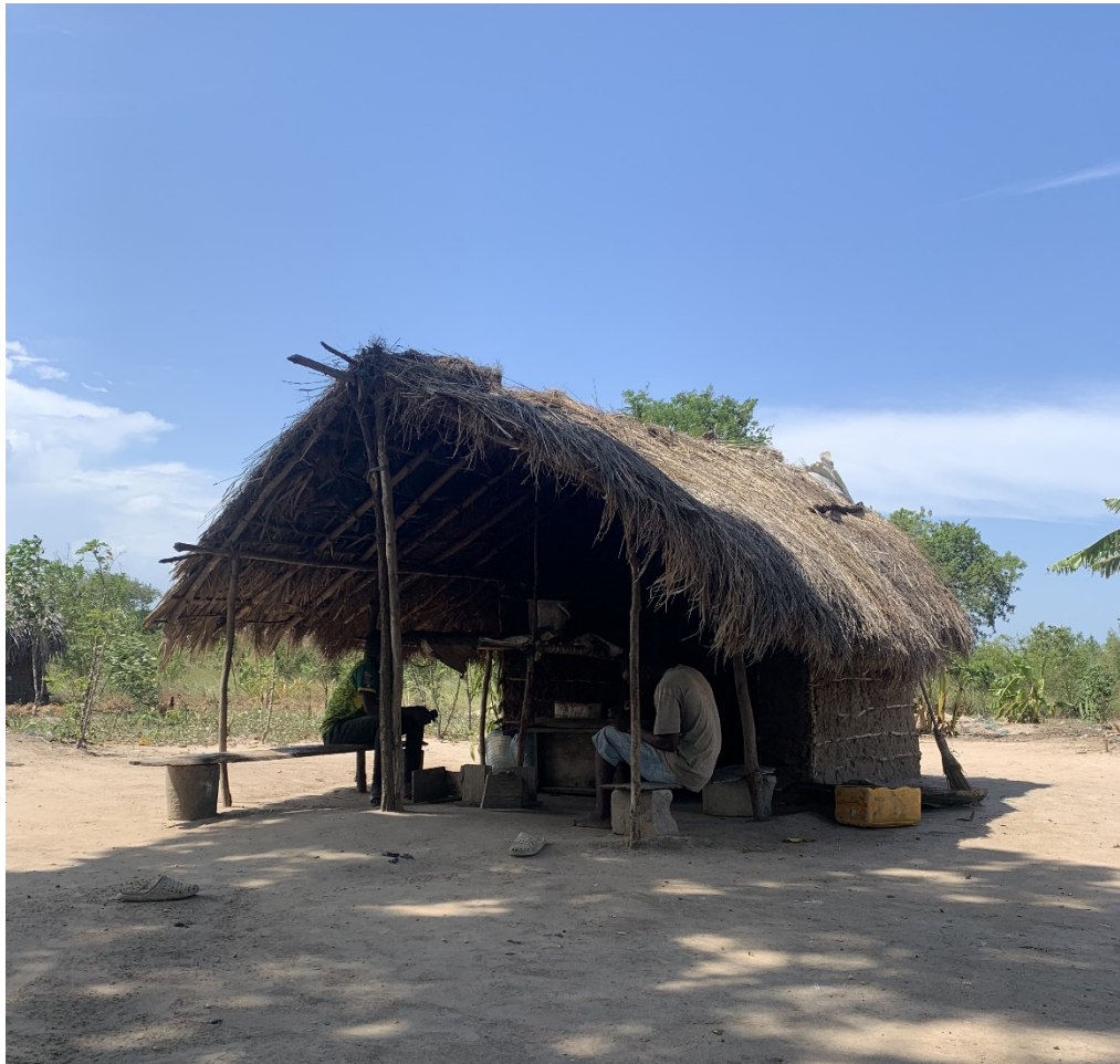
Figure 3: Clay house with thatched roof and wooden pillars. Photo taken by author. 10
