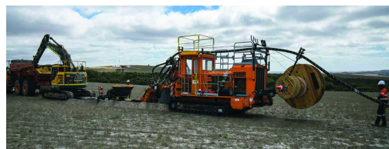
Figure no. 34 Cable laying process after levelling.
