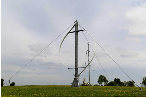
Figure no.12: Darrieus wind turbine.
