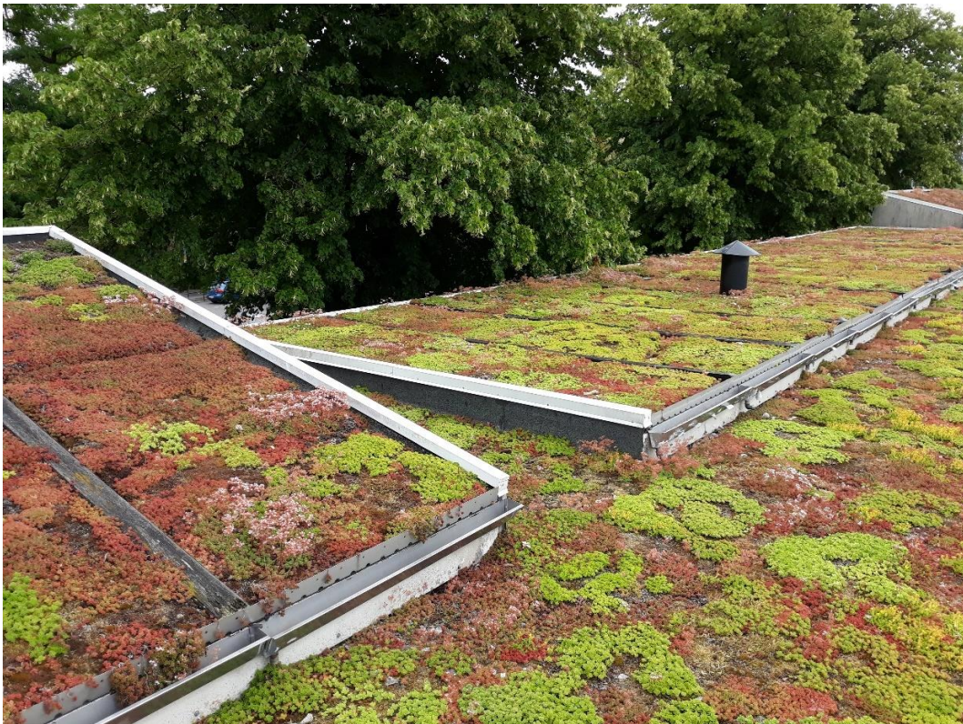
Figur 1. Sedum- mosstak. Foto: Green Roof Aging Project.
