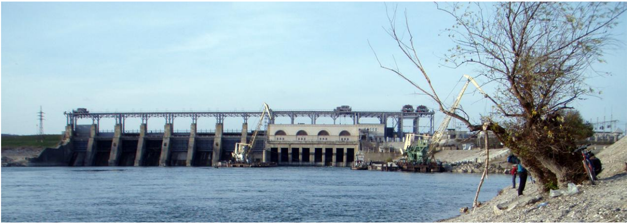
FIGURE 32: HYDRO POWER PLANT IN DUBASARI, TRANSNISTRIA. PHOTO TAKEN BY ANNELIE KJELLBERG
