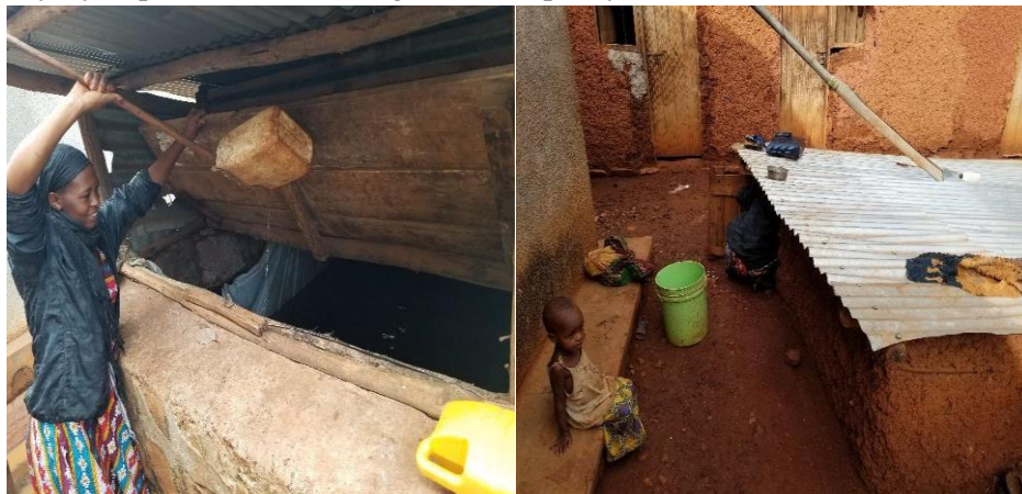
Figure 4. Underground tanks for rainwater harvesting, Gatore sector/KIREHE
