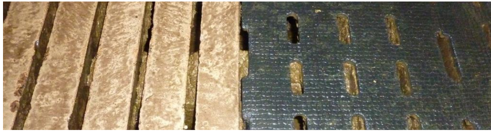
Figure 2. Slatted floor with and without rubber mats. Photo: Christer Bergsten.
