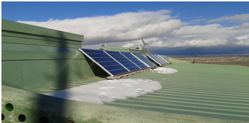
Figure 2. Solar panels on the rooftop of an Earthship. Taos, New Mexico, late December 2015.
