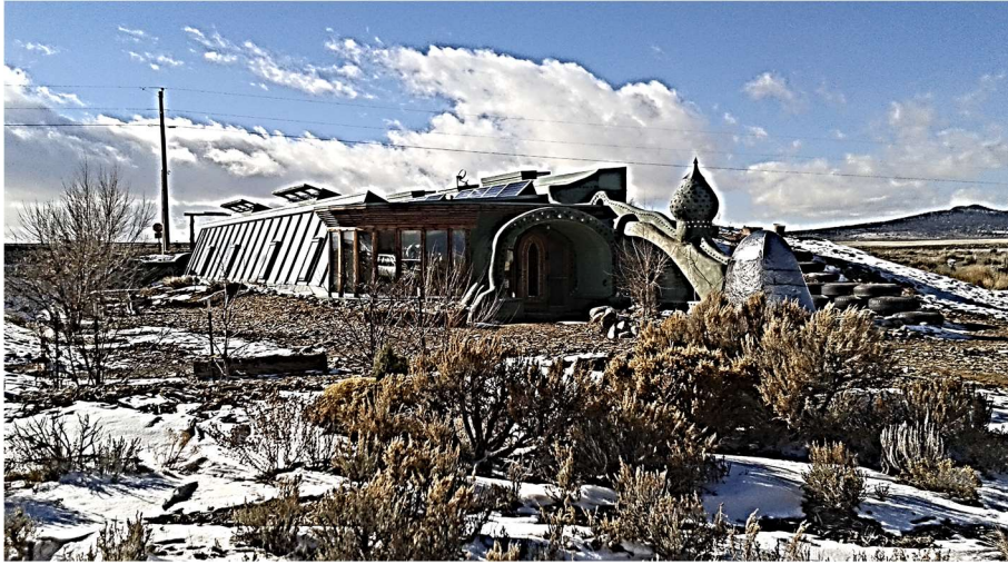
Figure 1. Earthship at the Earthship Biotechnology visitor center. Taos, New Mexico, late December 2015.
