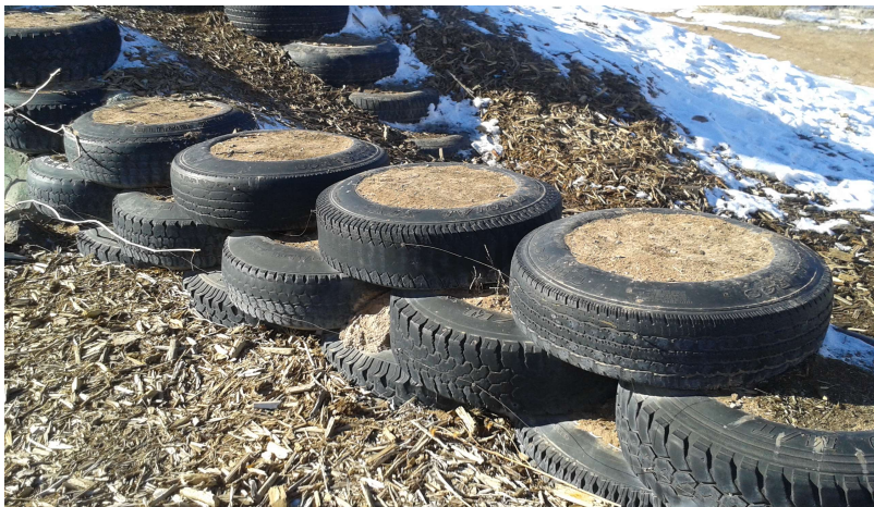
Figure 3. Stacked car tires rammed with earth. Taos, New Mexico, late December 2015.
