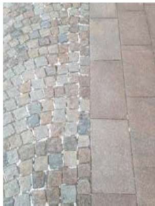
Figure 79. Bush hammered cobblestones.
