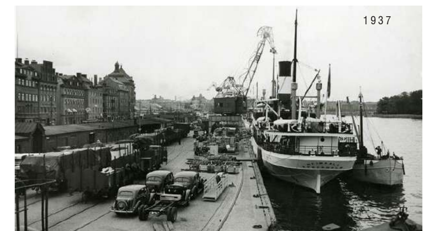
Figure 47. The photograph from 1937 show how cranes - rolling on tracks between quayside and customs houses un-/loaded the ships and carriages.
