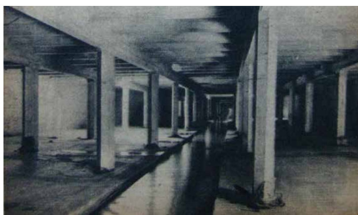
The second phase in the construction work started in 1929 and required a hundred of workers to rise columns to support the road Juan B. Justo Av
