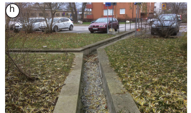
Fig. 33. Deep, concrete part of the drainage corridor.
