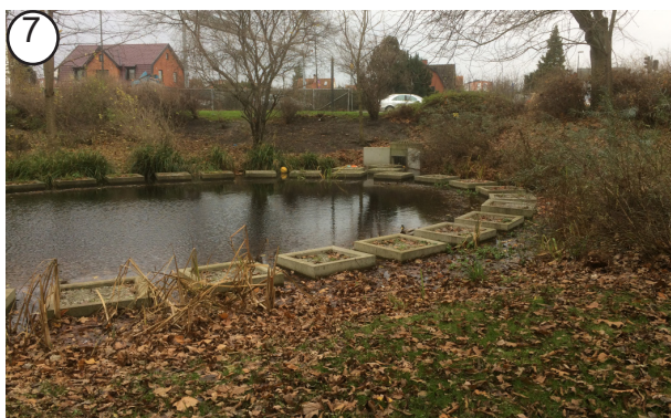
Fig. 23. Final step in the Central Drainage Corridor. When the water level is too high, the water passes through the opening at the end.
