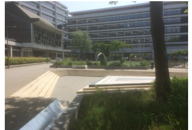
Fig. 51. One end station for directed water, led by steel gutter presented in down left corner.
