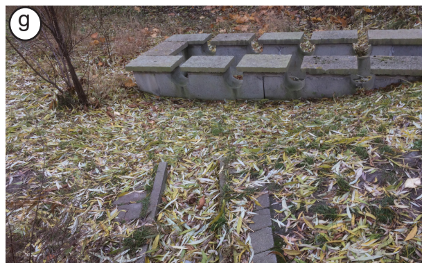
Fig. 32. Upwards elevated drainage channel. When the water reaches a certain level, it will pour through and into the drainage corridor.
