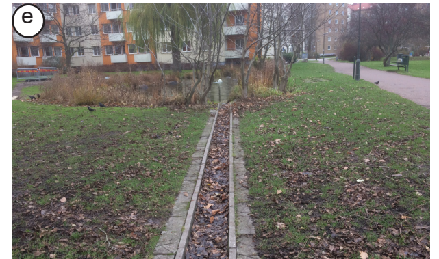
Fig. 30. Stormwater drainage within one of the housing areas.
