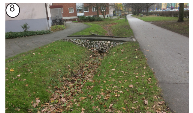
Fig. 24. Part of the Lönngatan Drainage Corridor.
