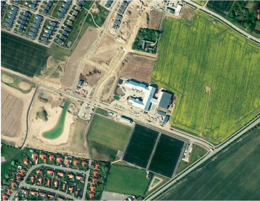
Figure 2. Aerial photo from eniro (eniro.se). In the middle of the photo is School 1. The school is located in a residential area with surrounding fields. Since this photo was taken more houses have been built next to the school. In front of the school there is a car road leading to the residential area. There are also football fields just outside the school ground, which belongs to the local football club.
