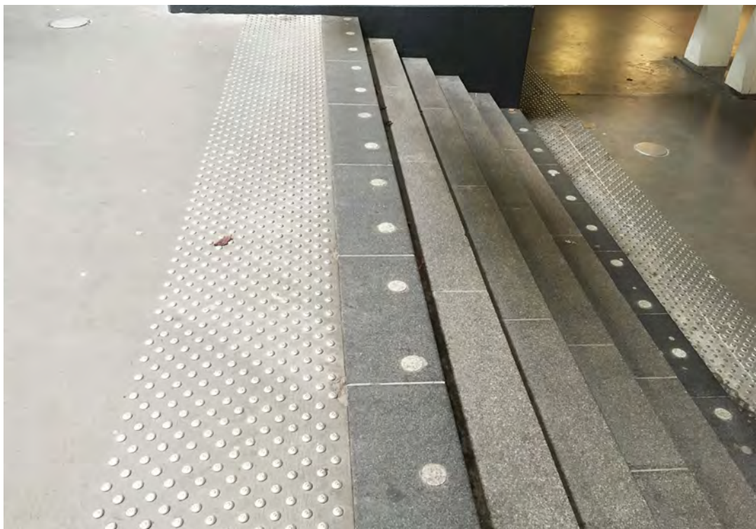
Figur 45: Pluggar i betongen
