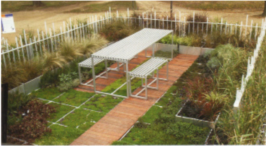
Fig 5.10 Extensive green roof and eating area on the 2005 Rhode Island School of Design Solar Decathlon House. (Picture: Jonathan Knowles, Kwok et al 2007, p. 50)
