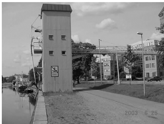
Figure 13 Silo port in Uppsala
