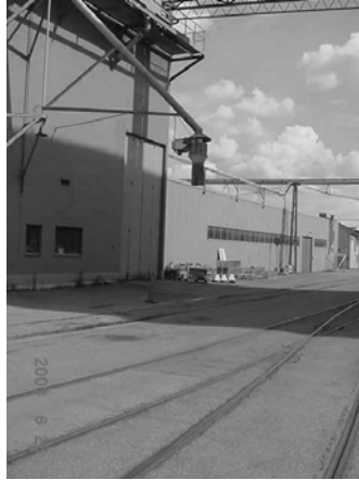
Figure 14 Loading facility for train and lorry at the Uppsala silo
