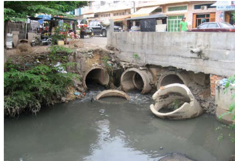
Degradation of drainage pipes due to neglect during the Khmer Rouge period. (Photo: Sara Rytter)
