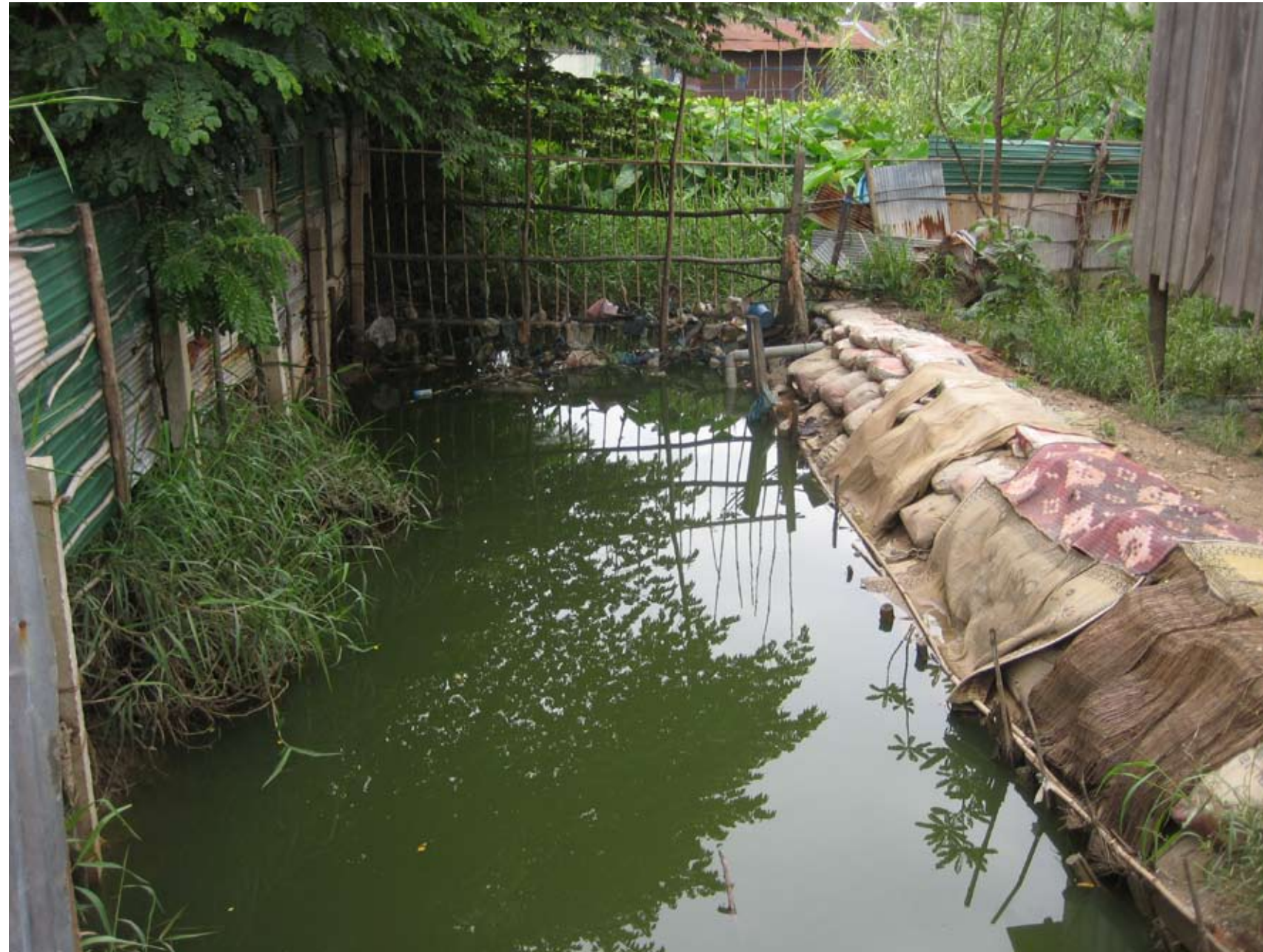
The northern canal leads surplus water from the Boeng Kak Lake to the Tonle Sap River. Sand bags are protecting the close by houses and land from the rising water levels during the rainy months. (Photos: Gunilla Englund)
