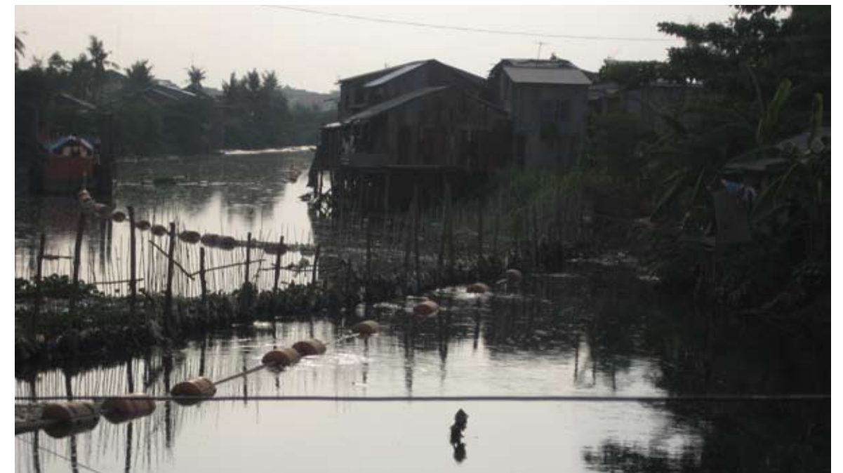
Trabek pumping station. Only a fence of bamboo bars prevents big pieces of garbage to flow into the pumps. The floating garbage is being collected and gathered by the workers every day. Close to the pumping station there is a dumpsite for the collected garbage. The municipality collects the garbage when the dumpsite is full, in average every four months. (Photo: Gunilla Englund)
