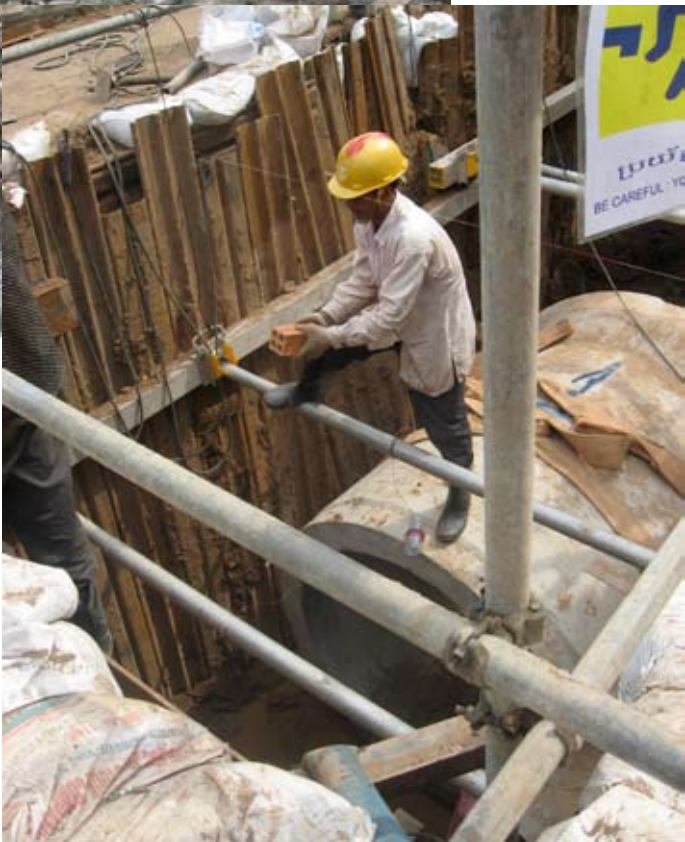
New drainage pipes replace the old and degraded ones. The work is ongoing in the most central parts of the city. (Photo: Sara Rytter)
