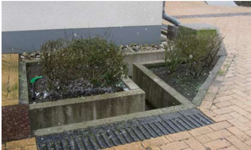
Storm water drainage in Bo01. The flower beds are not connected to the drainage system. (Photo: Sara Rytter)
