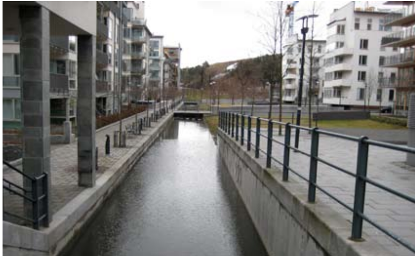
Main storm water canal in Hammarby Sjöstad. The canal has fixed concrete borders. (Photo: Gunilla Englund)
