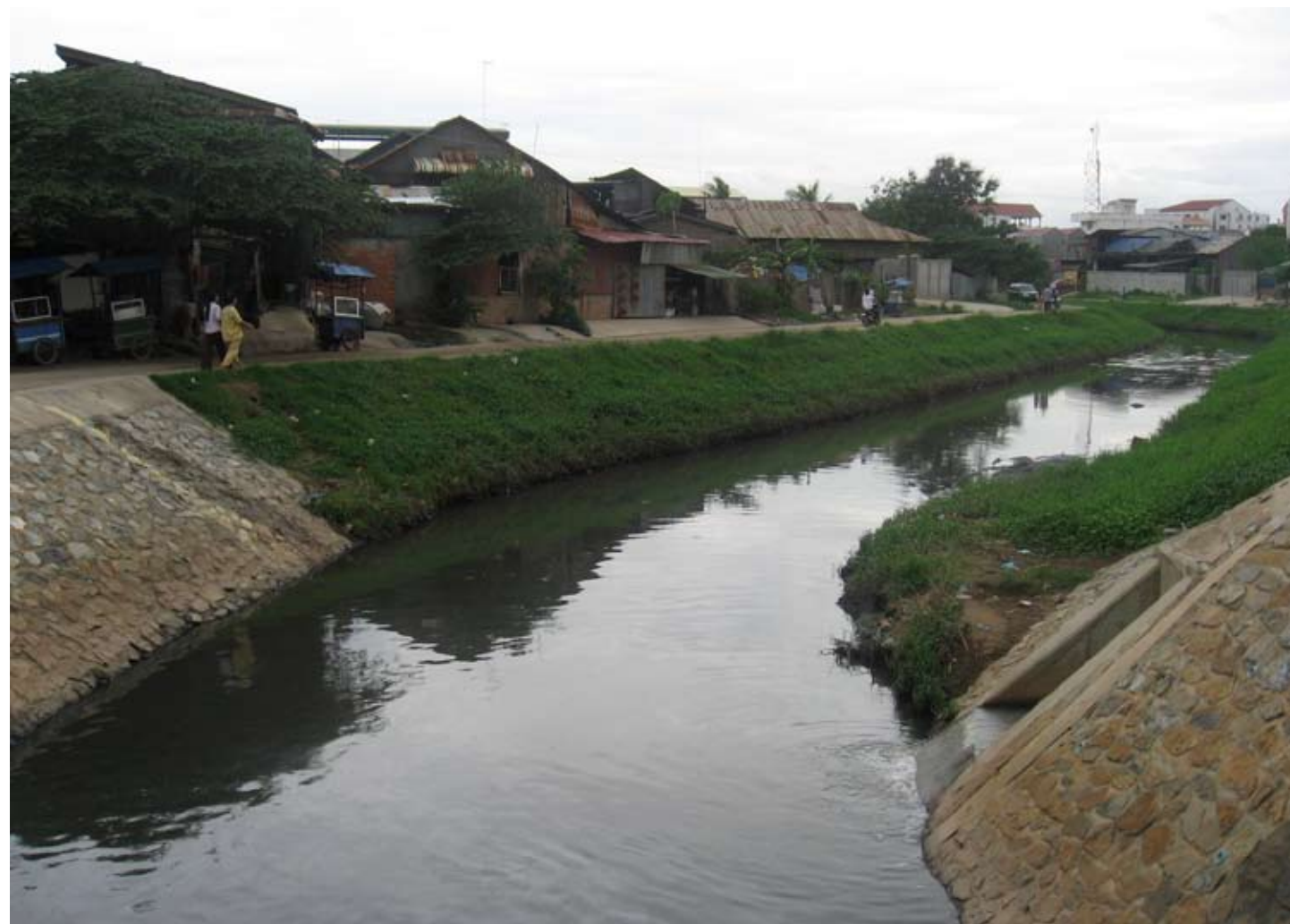
The restoration of the Salang Canal is partly finished. The part that is finished has sides of concrete and green areas where grass is established. New roads with sidewalks stretching along the canal are making it accessible for both private persons and garbage collectors. Before, slum settlers were living on the slopes, but they are now relocated. (Photo: Sara Rytter)
