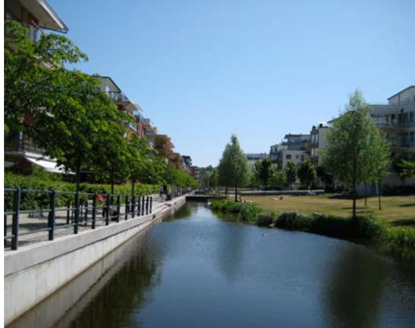
Storm water canal in the residential area Hammarby Sjöstad. During high water levels the water can flow over the green park area. (Photo: S. Rytter)
