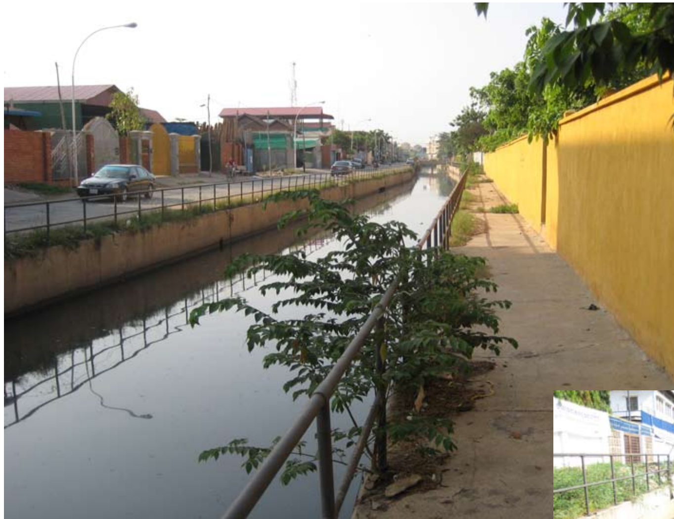
Trabek Canal has concreted sides to prevent erosion and flooding. (Photo: Gunilla Englund)
