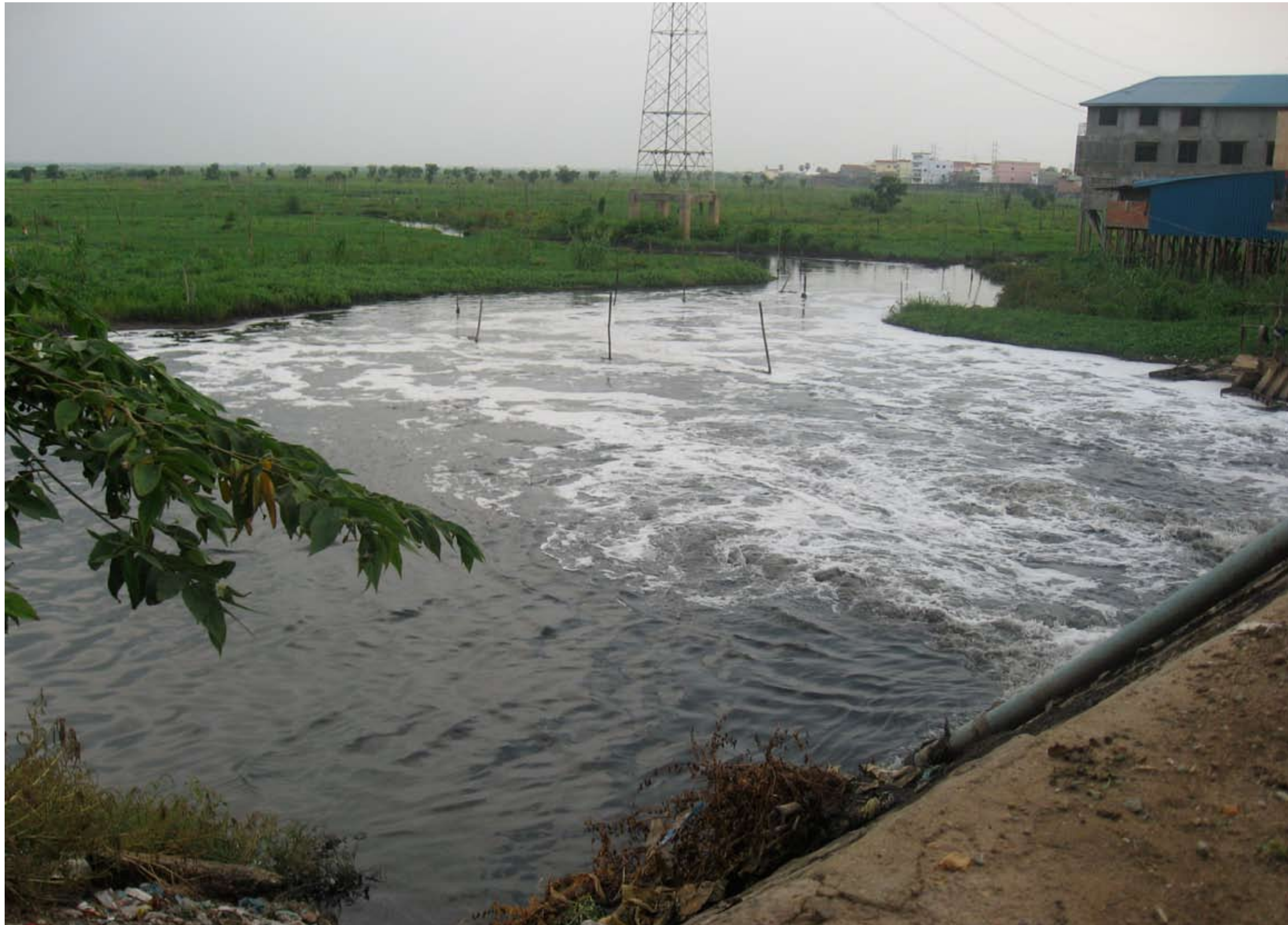
At the Trabek pumping station the water from Trabek Canal is being pumped over one of the road dikes (road 271) to the southern wetland. After the water has been pumped over the road it enters into the southern wetlands. It receives the majority of the city waste- and storm water. A couple of meters from where the untreated water is flushed out, vegetables are grown in aquatic cultivations and later sold on the central markets. (Photo: Sara Rytter)
