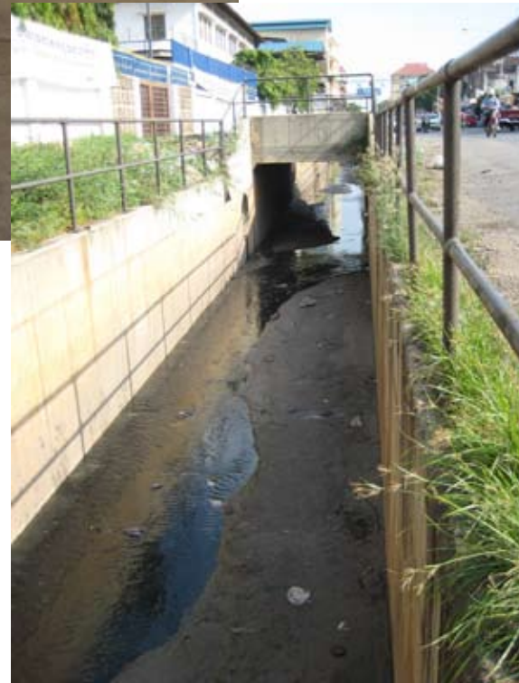
Sediments block the Trabek canal and reduce the water flow severely. (Photo: Gunilla Englund)
