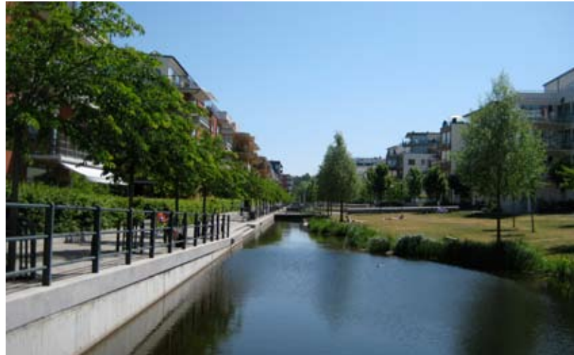
Main storm water canal in Hammarby Sjöstad. The vegetated surface gets inundated during heavy rain. (Photo: Sara Rytter)
