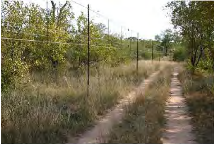
Figure 7. The partial enclosure.
