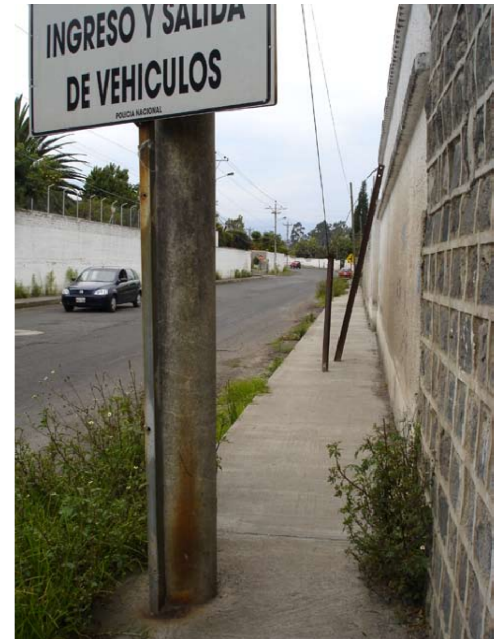
Unexpected hazards on the pavement in the streetscape defined by tall walls.
