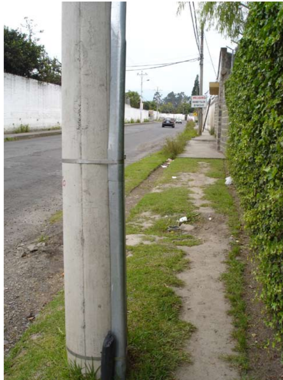
A green piece of pavement in need of maintenance.
