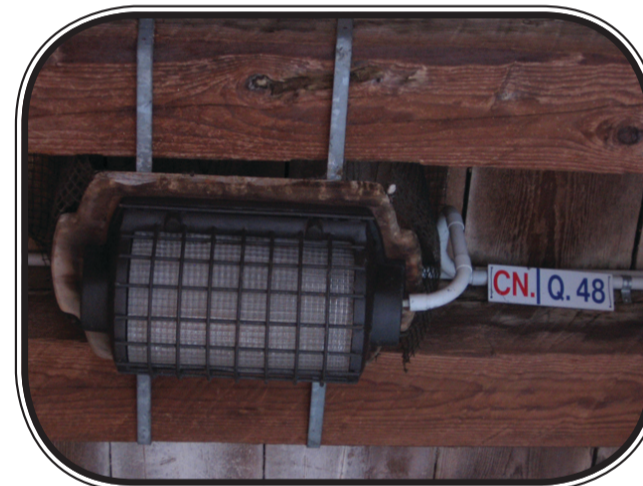
A robust type of luminary for the underpasses.
