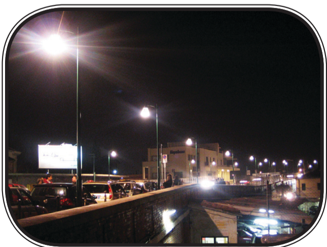
The existing lighting on the road to Piazzale Roma.
