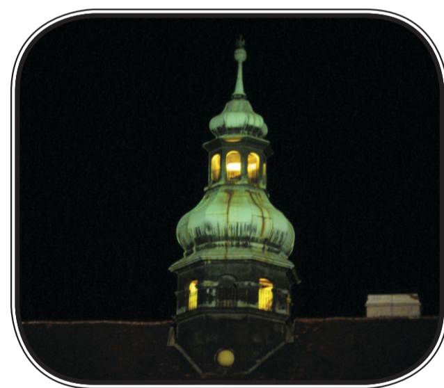
The top cupola of the church should be lit up in the same way but with a colder light colour..
