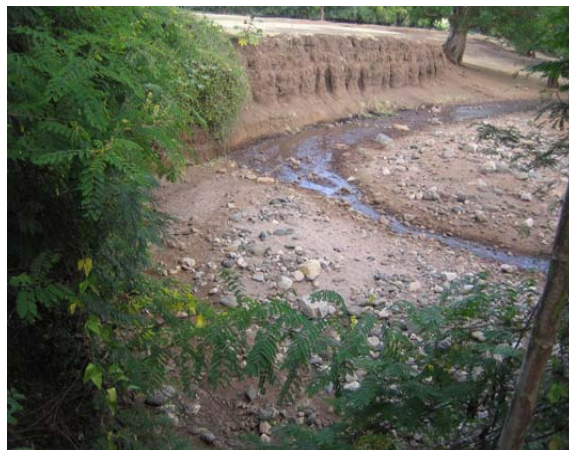
Fig. 7.2 Eroded river bank in Mamire ward.
