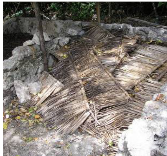
Fig. 4. The second compost compartment. During the two-month composting period, the ash and biodegradable waste are covered with makuti until ready for use as composting material in toilets.
