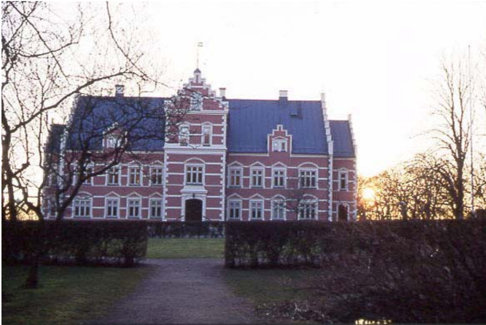
Figure 8. Pålsjö castle built around 1680.
