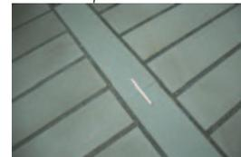
Fig. 93. Detail, Blue Stone with black sand stripes. Detail of the floor with Blue Stone and Black gravel. The decorative piece of metal in the middle is a handle used to reach structures below the paving.
