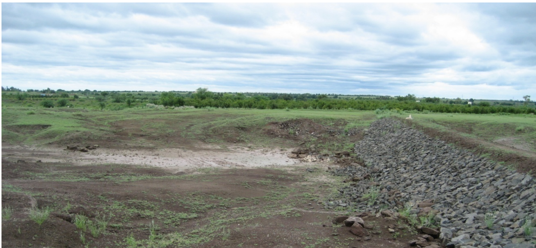
Figure 7.2 Check dam Flooding water coming from the left will stop when it reaches the dam wall. This allows more water to percolate through the ground.
