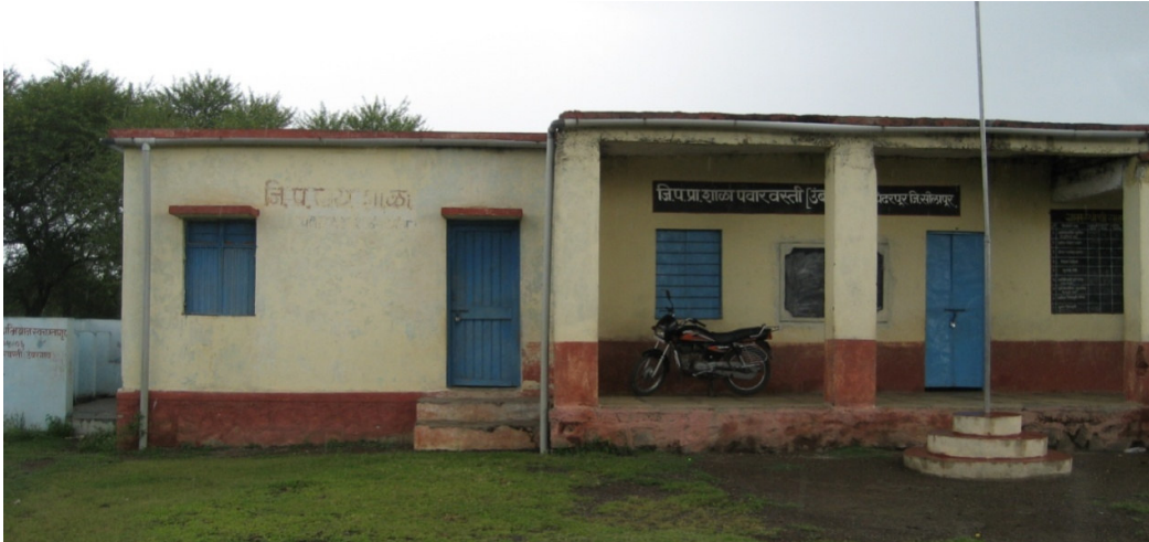
Figure 7.1 Roof rain water harvesting at a school The pipes leads water through a filter directly to the bore well.
