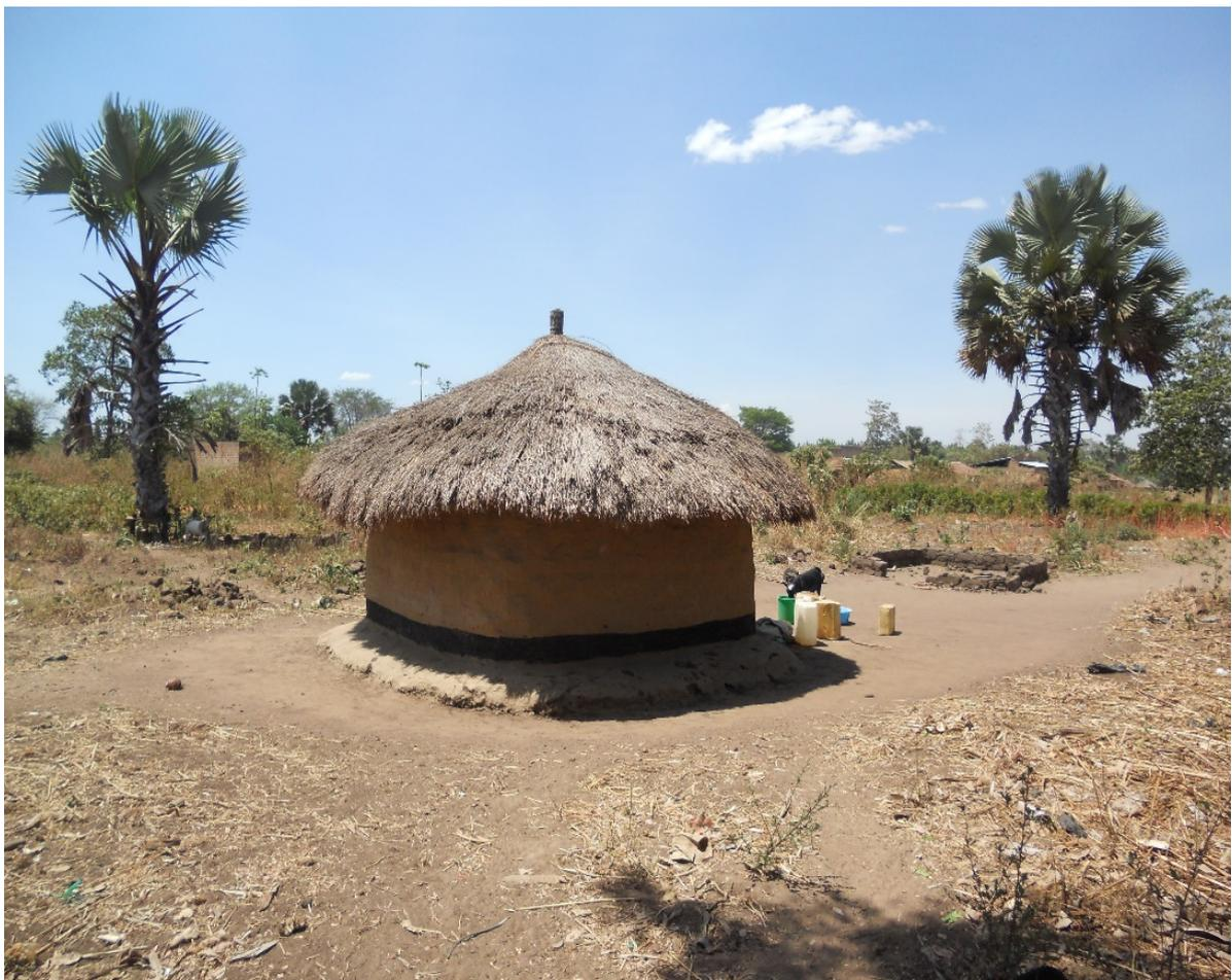
**Figure 4** Mud hut with grass-thatched roof.
