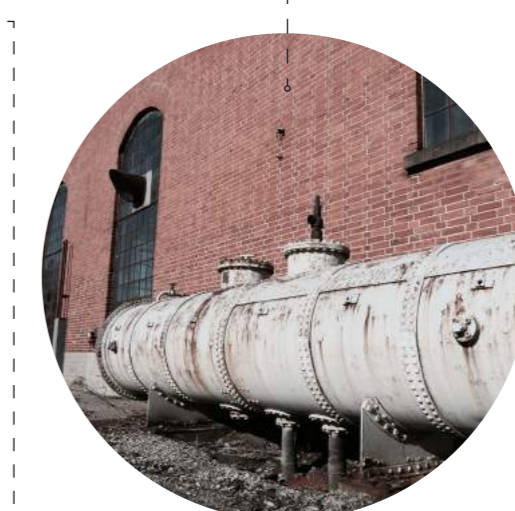
Tank invid restaurangfasaden
