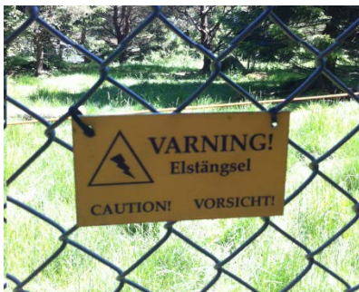
Figure 4. Proper signing of electric fence.
