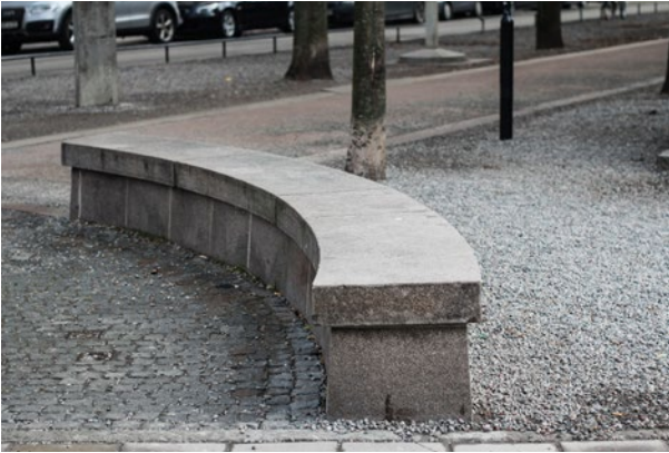
Cobble stones and gravel on each side of this otherwise perfect ledge has protected it from skate-related wear and tear without the use of negative design.
