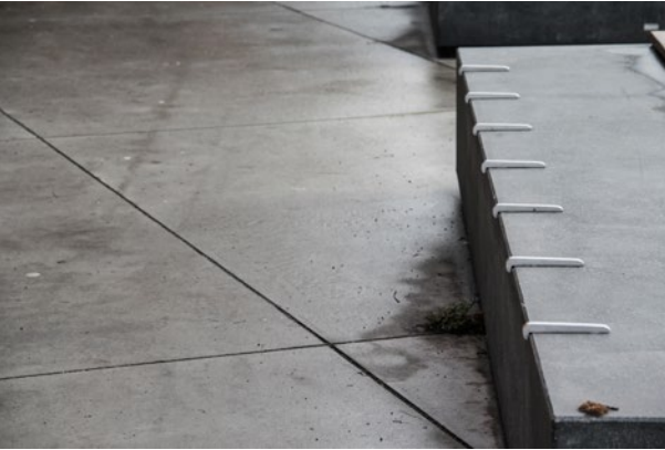
Skate stoppers save these fragile terrazzo ledges from skate-related wear and tear, but at what cost? Choose adequate materials.
