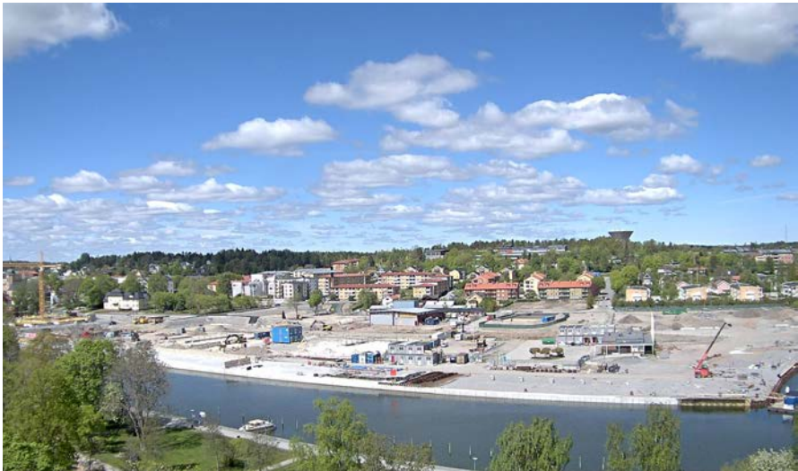
View showing the site, Norrtälje harbor, that is currently a construction site. Foto: Norrtälje hamn http://norrtaljahamn.se/webbkamera/ [2017-05-26]
