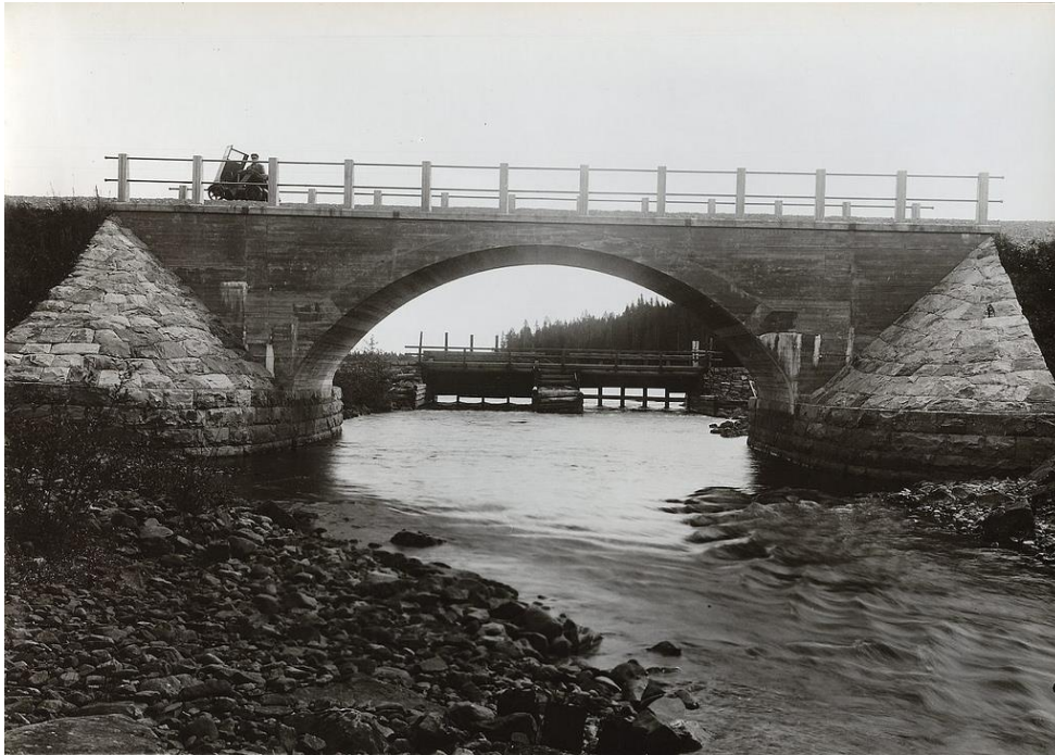
Figure 22: Railway bridge over Horrmundsvallen and the regulating dam by Lake Horrmunden. A person with dresin, picture taken around 1915 (Flickr, Tekniska Museet, 2015)
