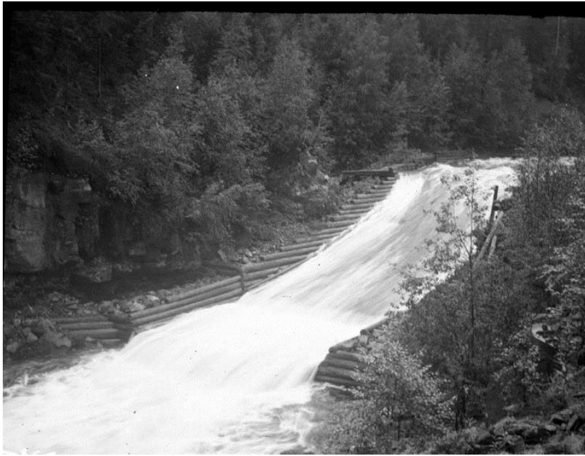
Figure 19: Horrmundsvallafallet, the fall is affected by the log driving activities. A weir has been constructed to make the log driving easier. Stones have been placed in the timber constructions. The picture is taken 1915-07-29 (SMHI, historiskt bildgalleri, 2015).
