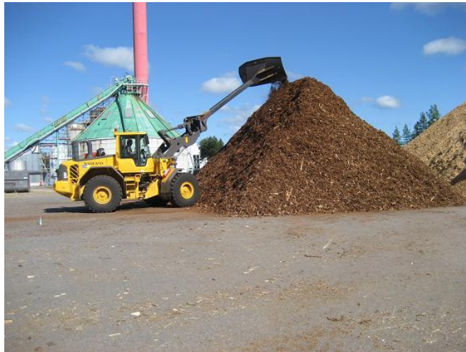
Figure 4.1, Johannes combined power and heating plant in Gävle, Sweden
