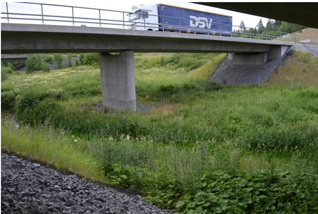
Fig. 3. The underpass with water and vegetation west of the wildlife passage. (Photo: Johnny de Jong)
