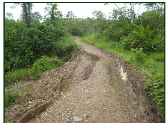
Illustration 16: Two months after the flooding, landslide
