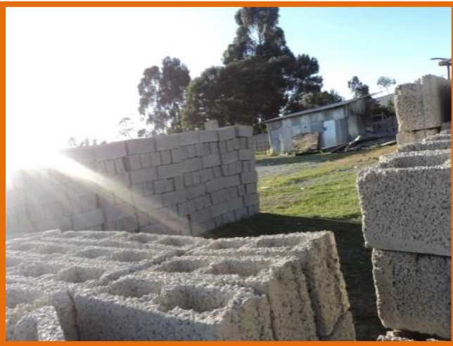
Figure 13 HCB construction on local open space
