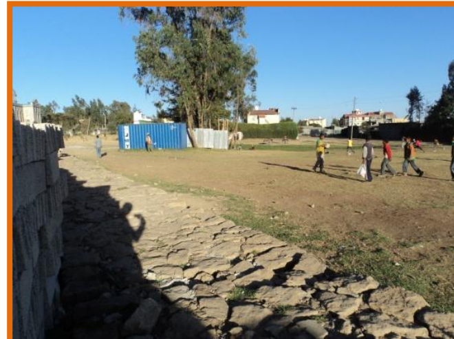
Figure 14 children playing along HCB construction
