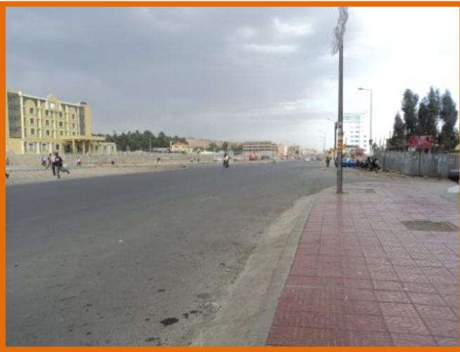
Figure 20 Wide street with empty side walk
