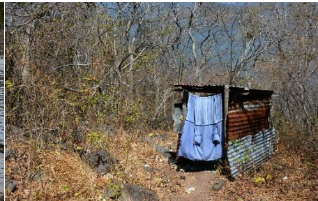
Figure 10. A typical pit toilet in El Morro.
